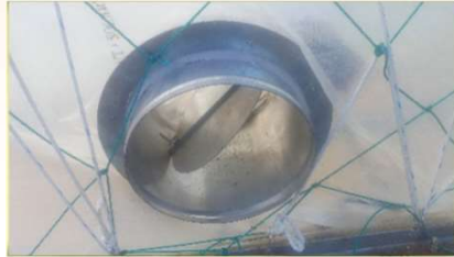
Hot air outlet (ceiling)
