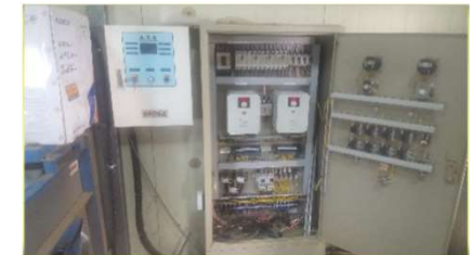
Temp/Humid Control unit
